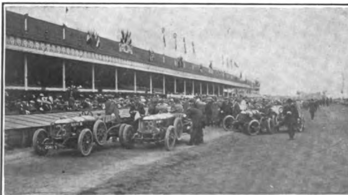
General view of the start and portion of grand stand
